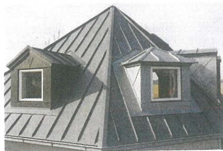
FIGURE 9.5.2 An aluminium window frame is resistant to corrosion and is a useful material in situations where maintenance would be difficult.
